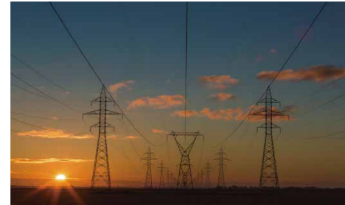
Power Line Inspection
